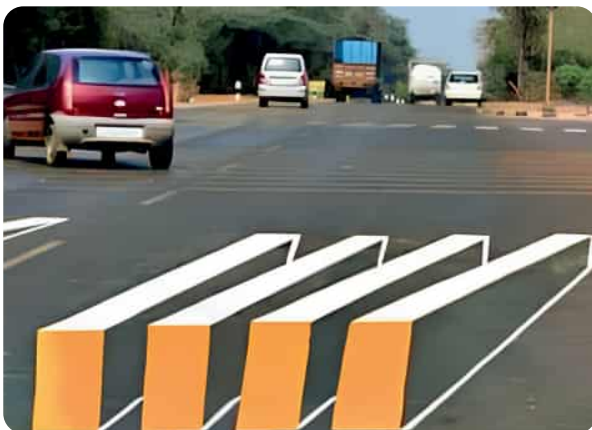
Figure 19: Zebra crossing installations in Bihar
