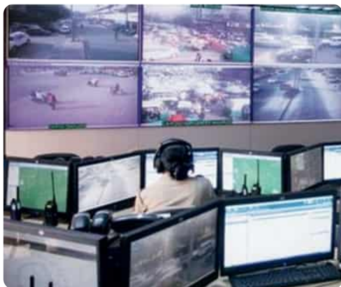
Figure 32: Command and control centre for VLTD, Himachal Pradesh
